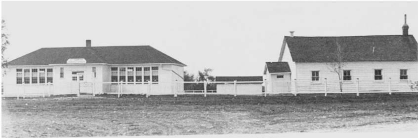
Original St. Andrews School (logs covered with siding) and new school, approx 1937.
