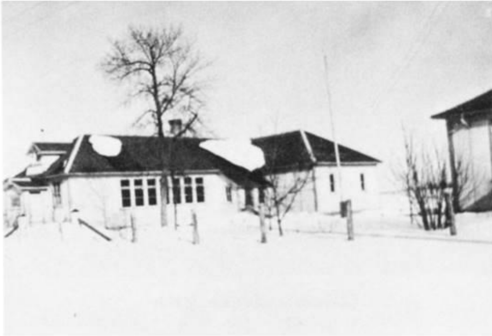
Donald School North and South Buildings
