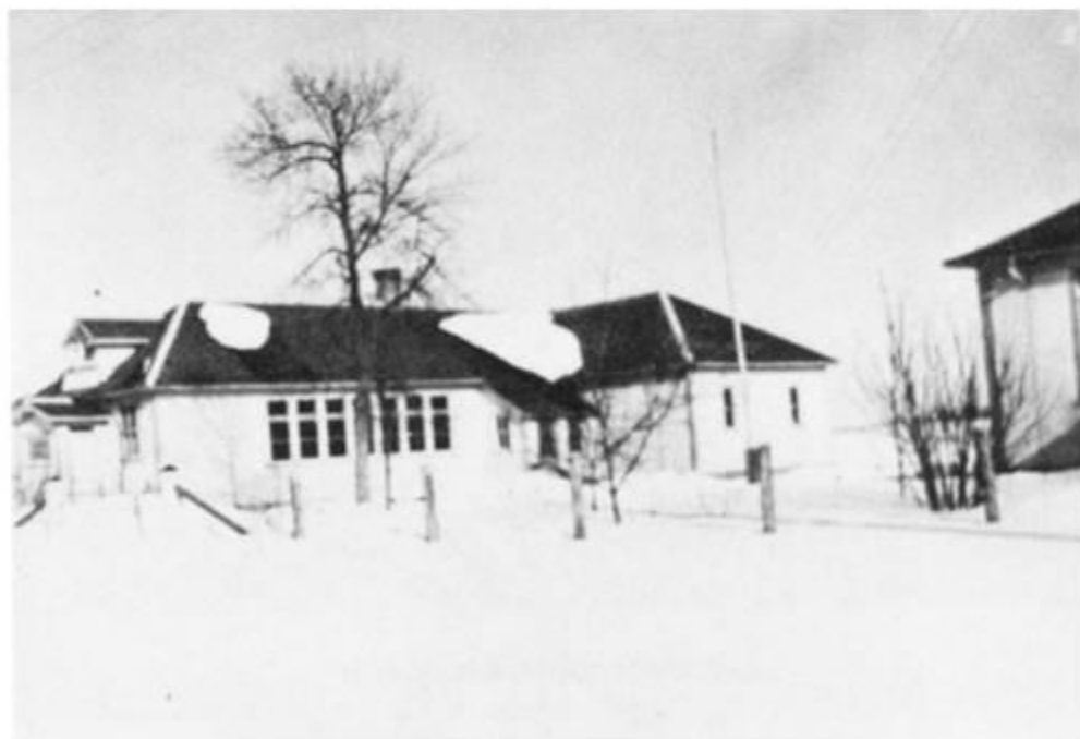
Donald School North and South Buildings
